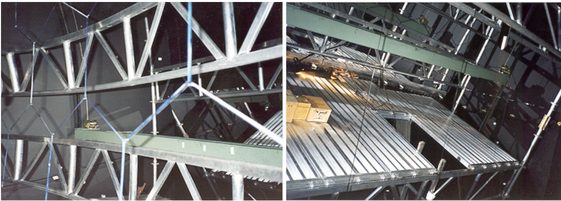
Figure 4.5: Spherical (left side) and planar (right side) mirror plane layout before the scaffolding was removed.
